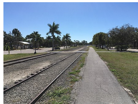
Seminole Gulf track through Downtown Bonita Springs. The platform is all that remains of the Atlantic Coast Line's passenger depot.
